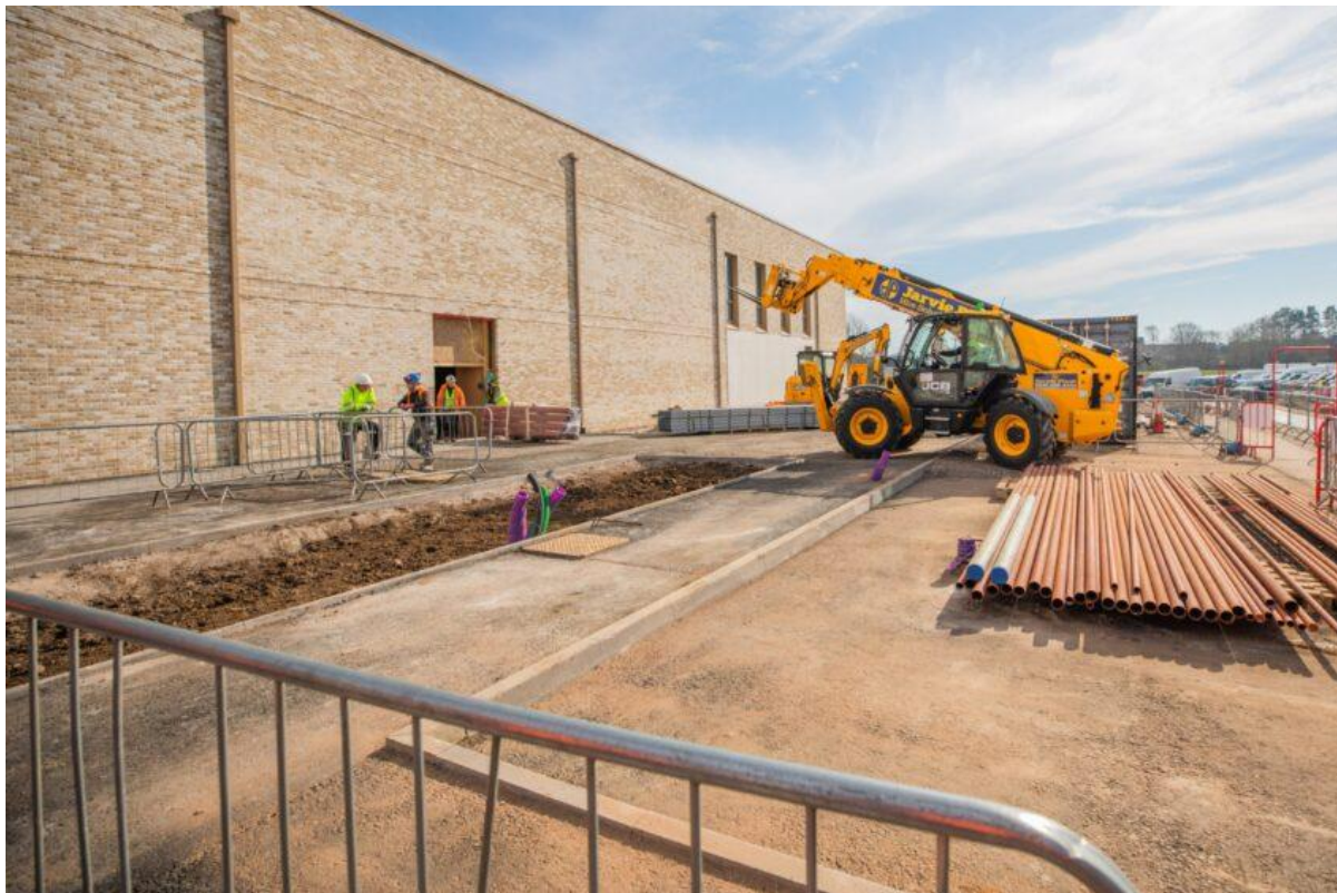
Diggers are still busy at the site.
